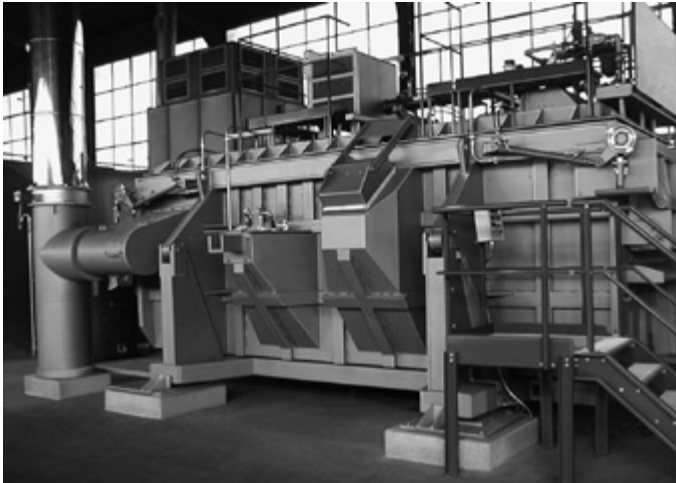
Aluminium industry: smelting furnace
