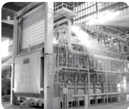
Bogie hearth forging furnace
