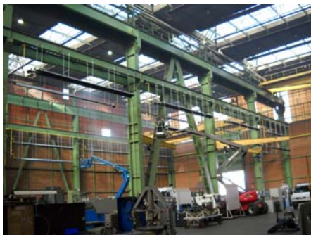
Gasgestookte donkere stralingsbuizen in "U", in lijn, in banen of in netwerk
