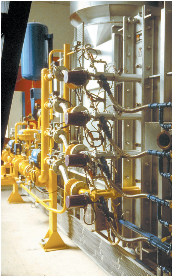
FlueFire system installed in a cogeneration plant
